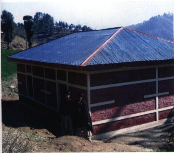
Hands-on training was given through the construction of earthquake resistant model houses for the most vulnerable households
